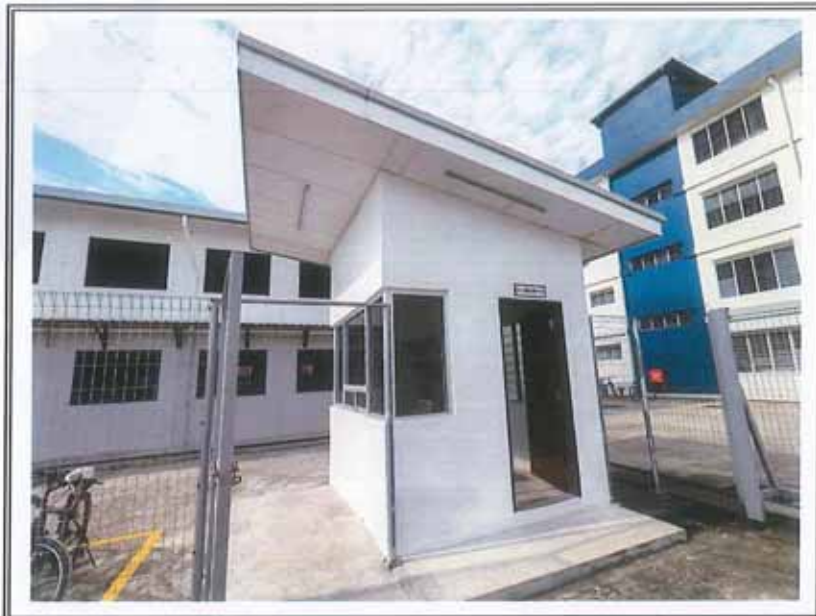
VIEW OF THE GUARDHOUSE 1
