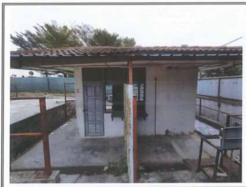
VIEW OF THE GUARDHOUSE
