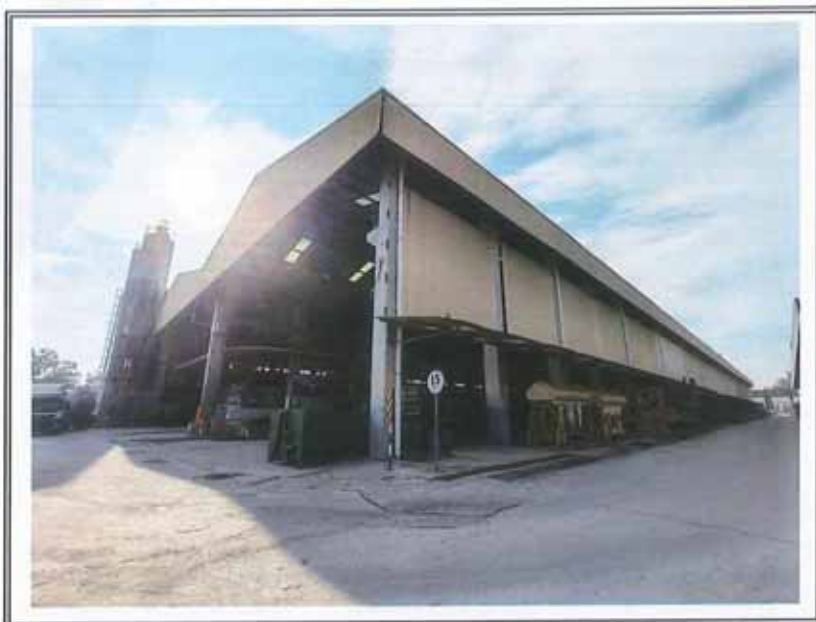
VIEW OF THE SINGLE STOREY OPEN SIDED FACTORY
