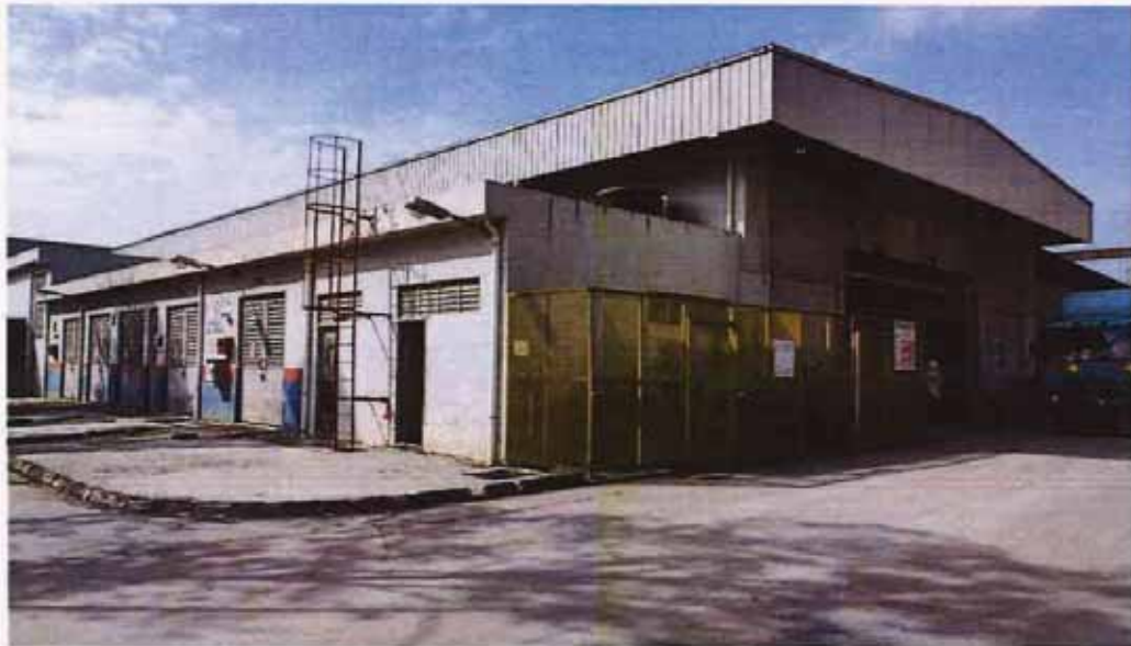
SINGLE STOREY WORKSHOP cum TNB-SUBSTATION
