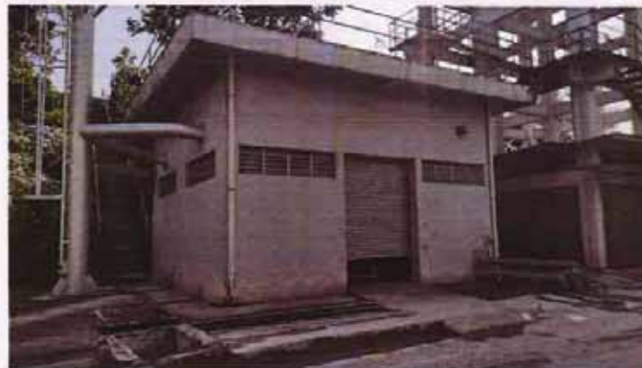
TWO UNITS OF BOILER ROOMS
