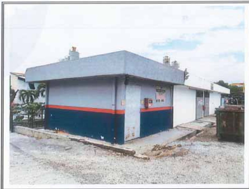
VIEW OF THE TNB SUB-STATION
