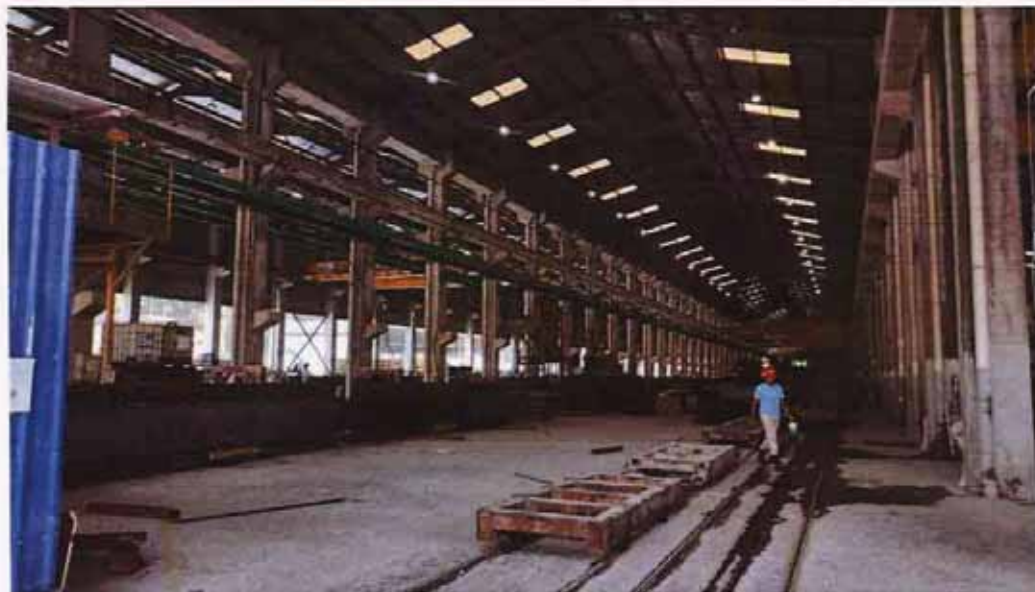
FOUR ADJOINING BLOCKS OF SINGLE STOREY PLANT BUILDING
