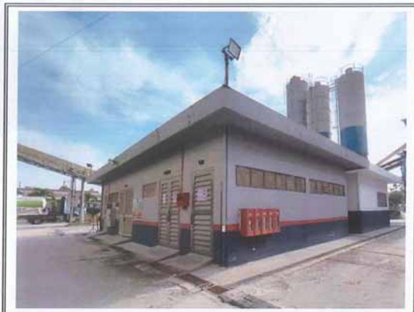
VIEW OF THE TNB SUB-STATION
