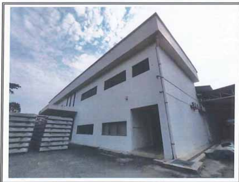
VIEW OF THE DOUBLE STOREY OFFICE BUILDING (OFFICE B)
