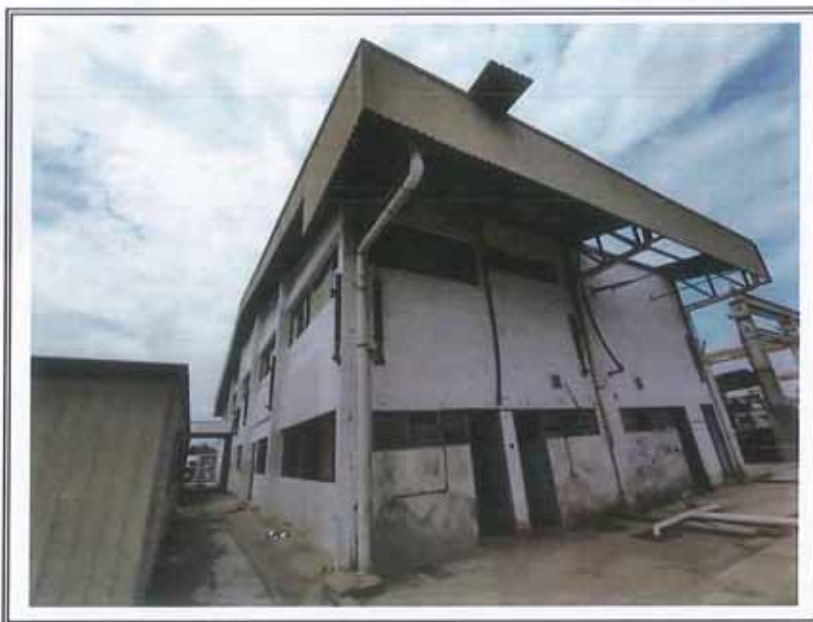
VIEW OF THE DOUBLE STOREY OFFICE BUILDING
