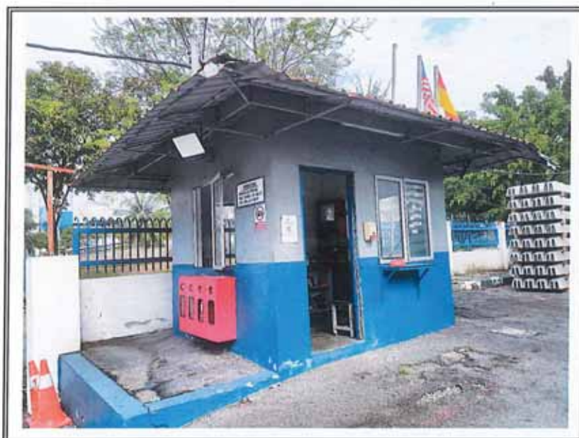
VIEW OF THE GUARDHOUSE
