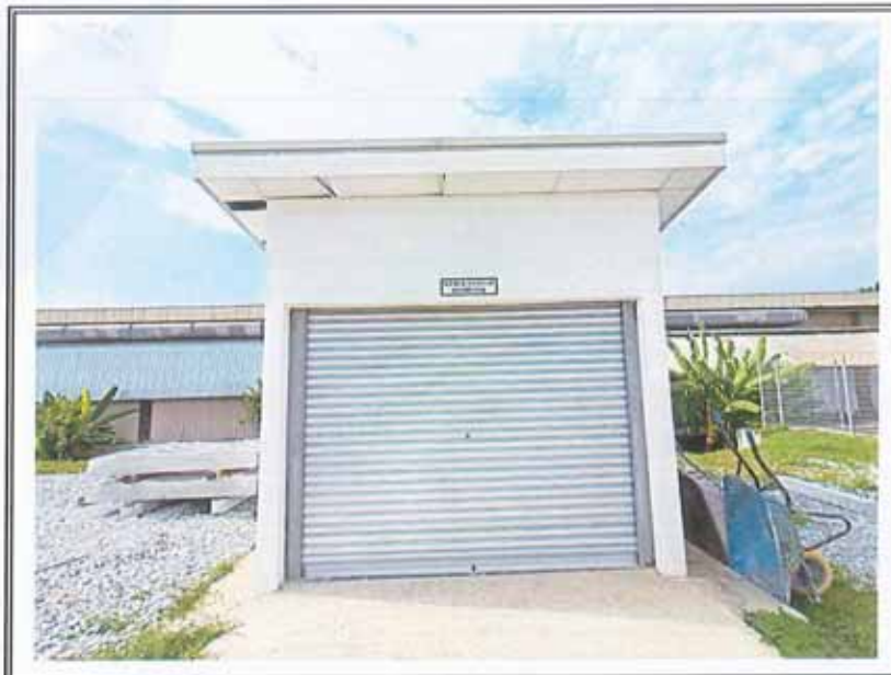
VIEW OF THE REFUSE CHAMBER
