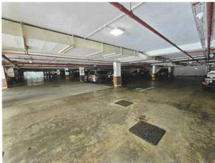
Annex Block – Multi-Storey Car Park
