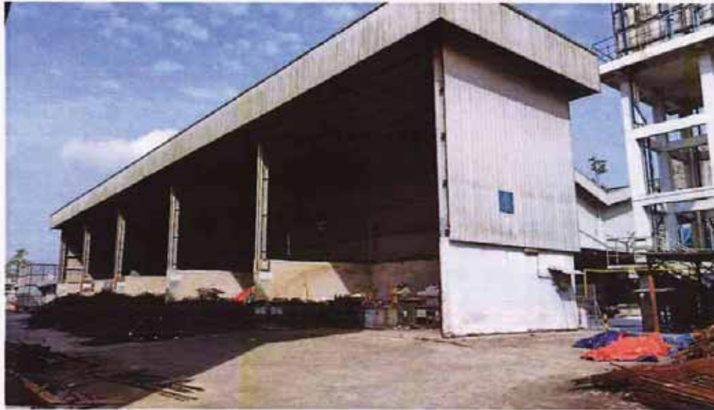
SINGLE STOREY SCRAPE METAL STORAGE
