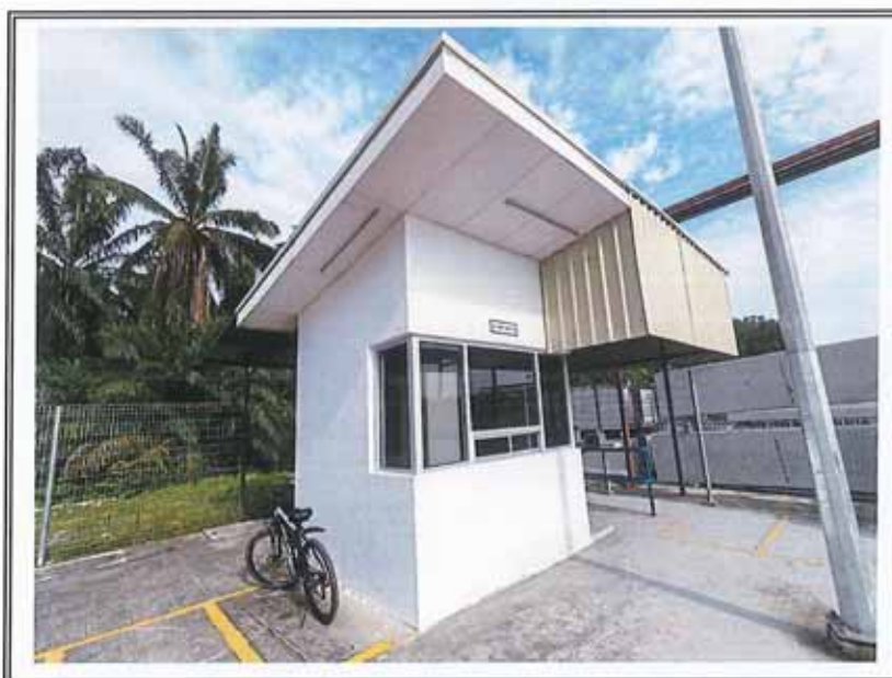
VIEW OF THE GUARDHOUSE 2
