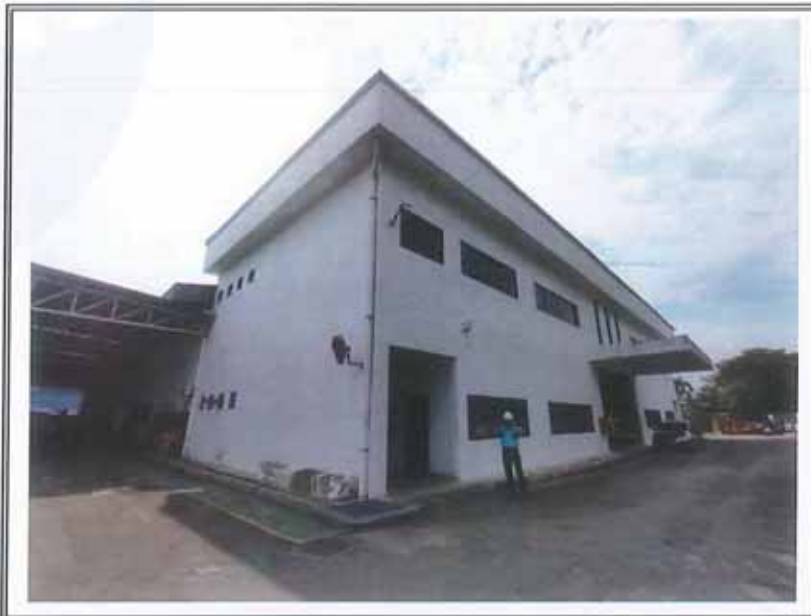
VIEW OF THE DOUBLE STOREY OFFICE BUILDING (OFFICE A)
