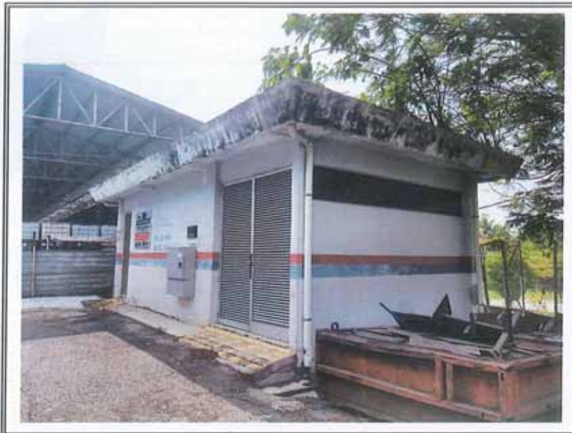
VIEW OF THE TNB SUB-STATION
