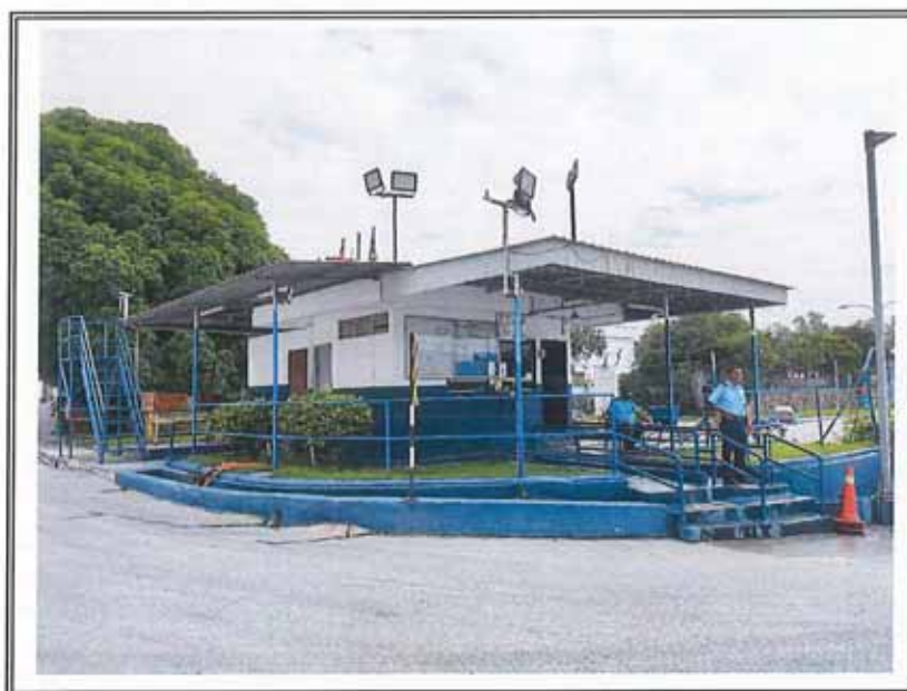
VIEW OF THE GUARHOUSE
