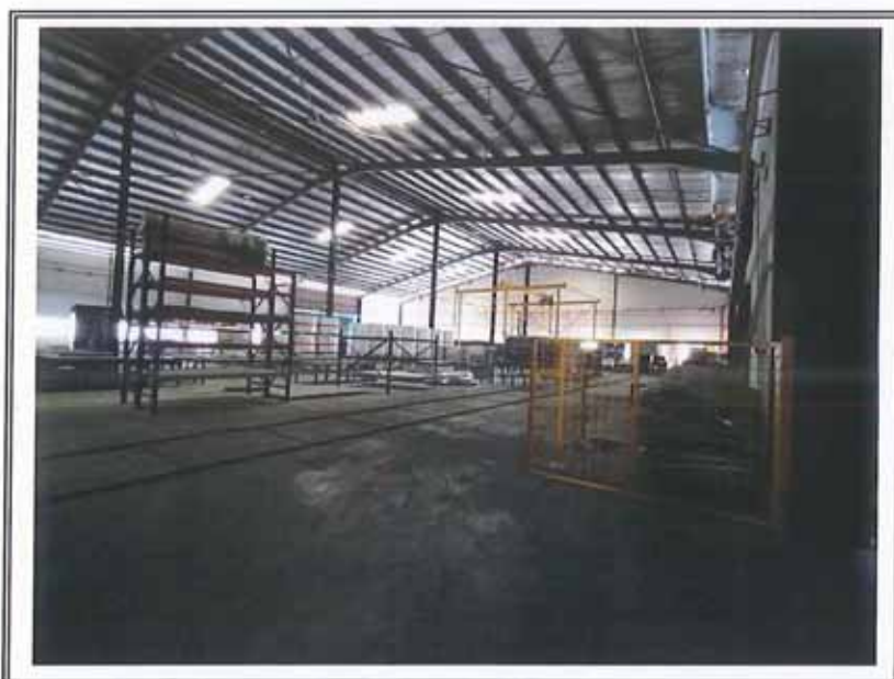
VIEW OF THE SINGLE STOREY FACTORY ANNEXED (FACTORY B)
