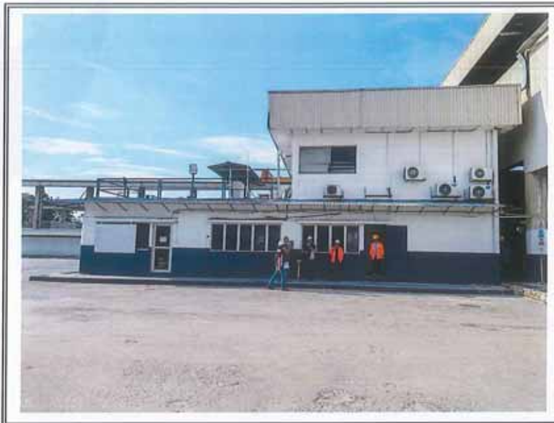
VIEW OF THE ONE-AND-A-HALF STOREY OFFICE BUILDING
