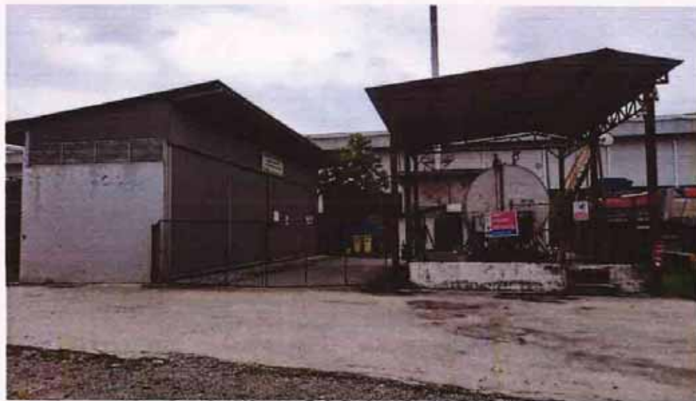
DIESEL TANK & SCHEDULE WASTE STORAGE
