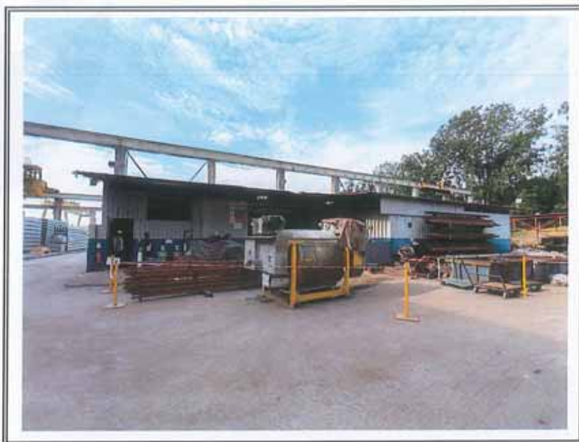
VIEW OF THE SINGLE STOREY WORKSHOP
