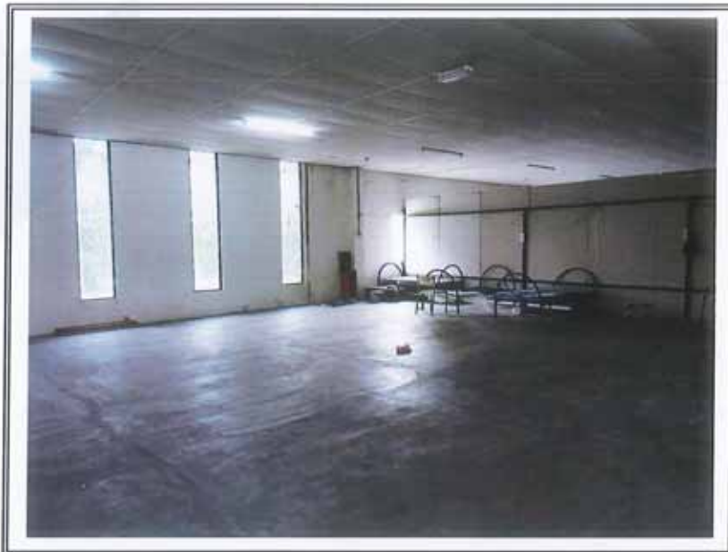
VIEW OF THE OFFICE AREA (OFFICE A)
