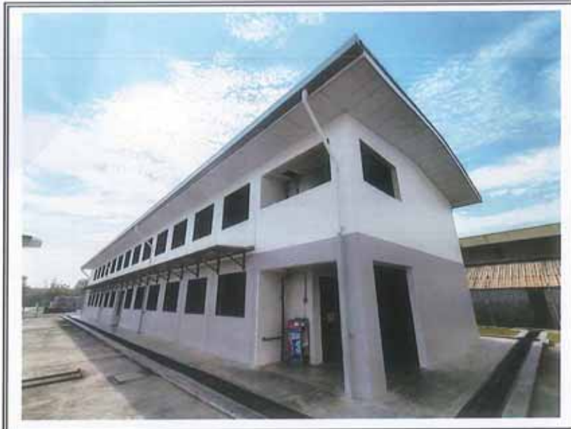
VIEW OF THE DOUBLE STOREY KITCHEN & DINING
