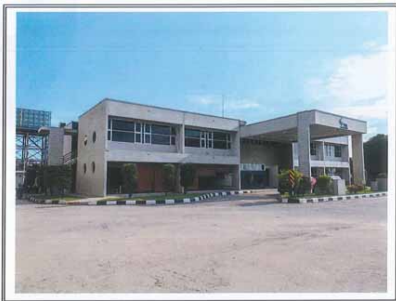
VIEW OF THE DOUBLE STOREY OFFICE BUILDING
