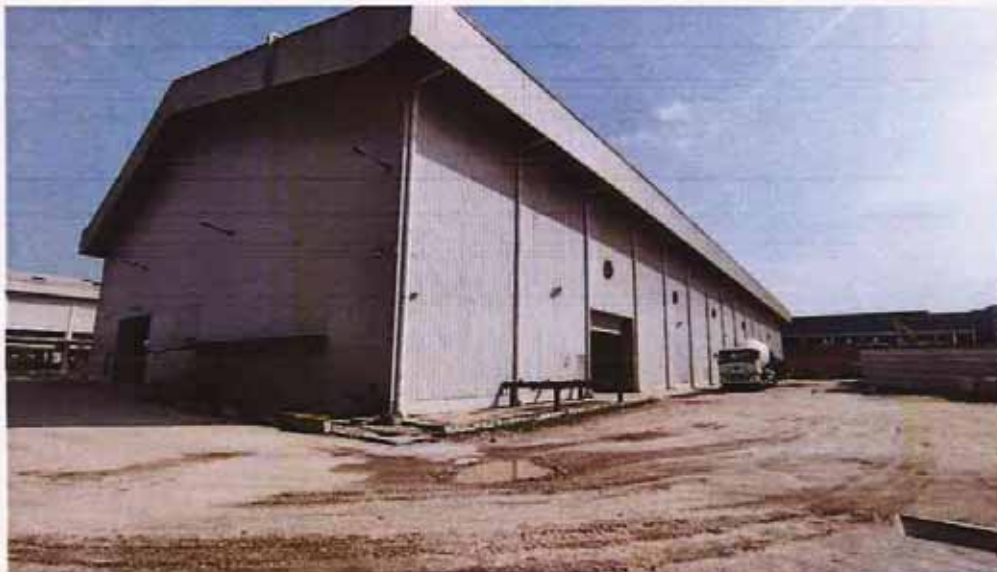
GENERAL VIEW OF THE SINGLE STOREY WAREHOUSE
