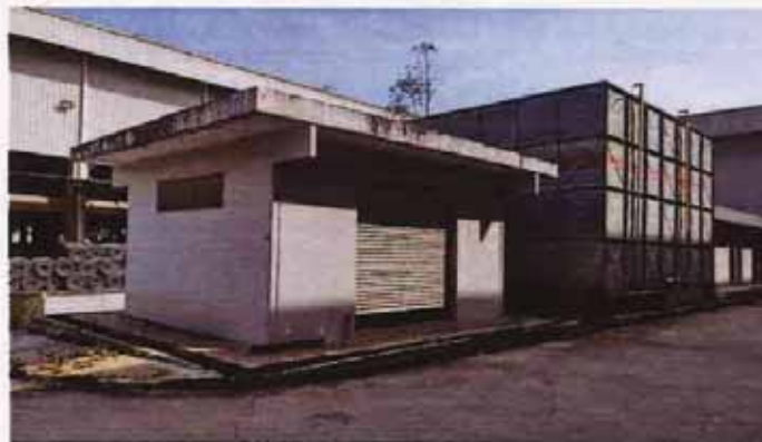
COMPRESSOR & PUMP ROOMS
