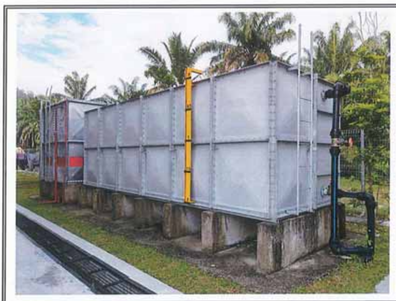
VIEW OF THE WATER TANK
