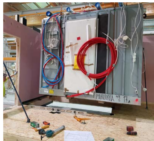
Unit bathroom in a module
