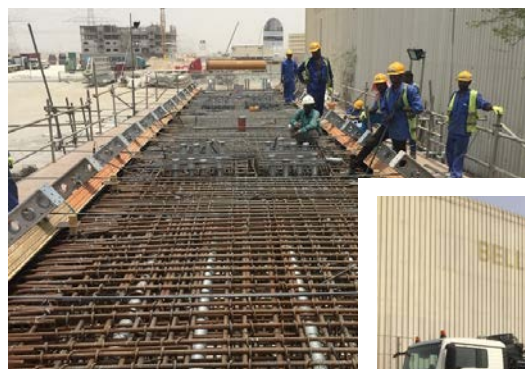
Workers casting for precast portal concrete beams
