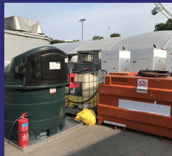
Harlequin tank supplying multiple Aggreko generators
