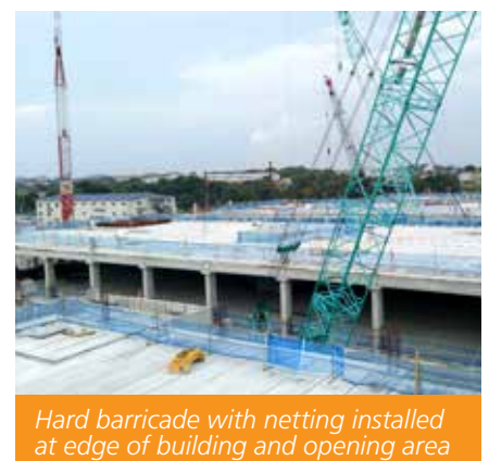
Hard barricades installed at site
