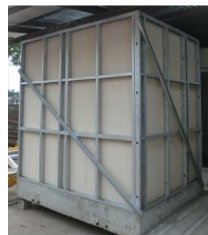
Metal frame PBU with drywall panels
