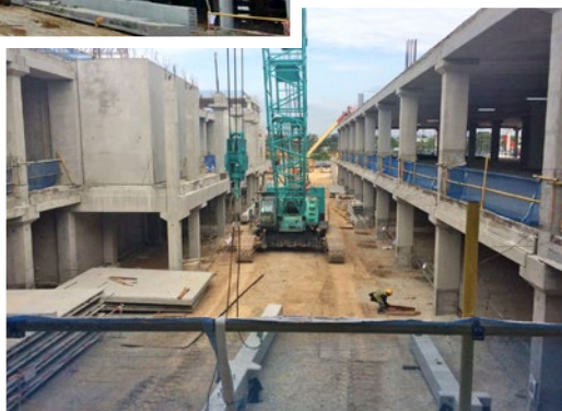
▶ Installation of massive 38 tonne precast beam
