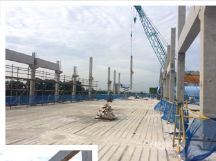
▲ Installation of precast columns to roof level
