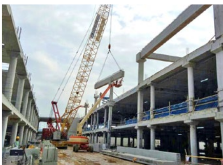
▲ Installation of precast columns to roof level
