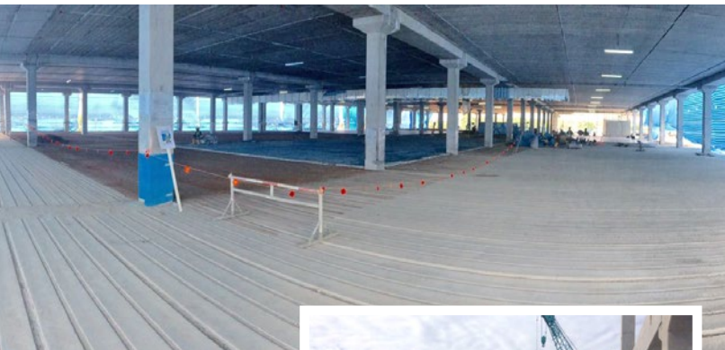
▲ Completed hollow-core floor ready for finishing works
