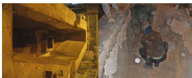
Checking of the lining after de-moulding
