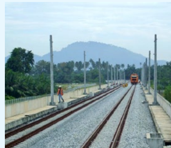
Railway Sleepers at Perak railway track
