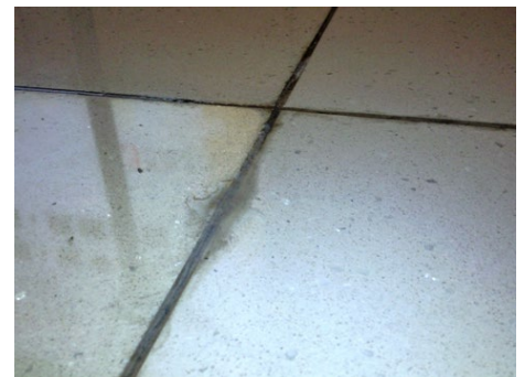
Signs of water spillage at grout areas
