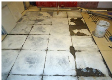
The floor tiles deformed and de-bonded from the floor substrate.
