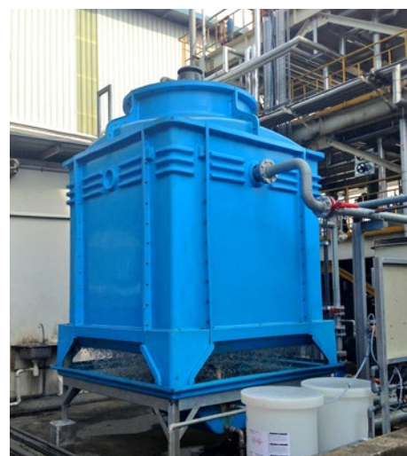
Cooling tower that reduces overall operating cost
