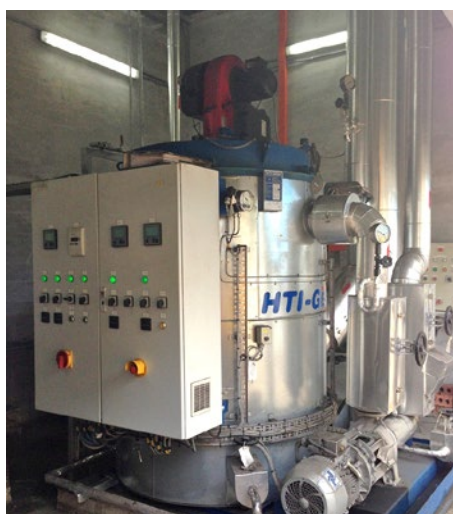
Newly installed diesel firing boiler helps to save cost
